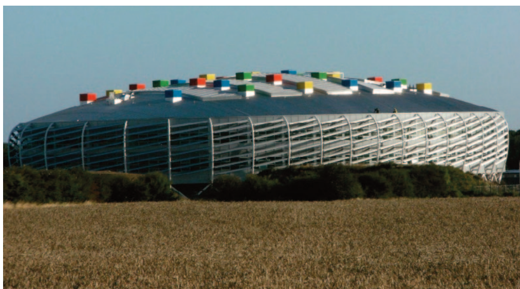
Example of building designed for Monkseaton High School (Newcastle) with ventilation provision being considered from the outset and e-stack units atop the roof. Photo courtesy of Breathing Buildings.
